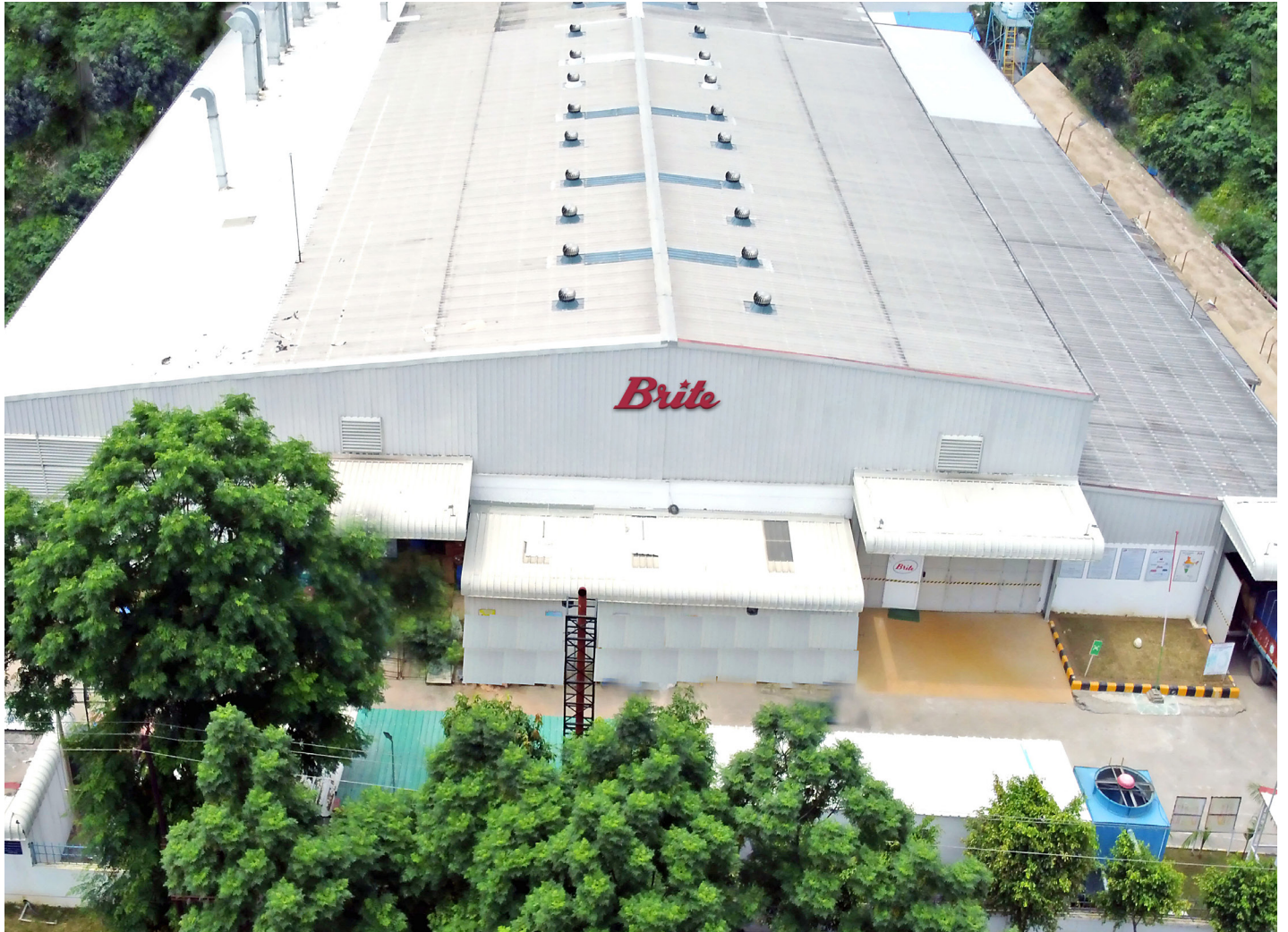
New manufacturing unit at SIDCUL, Haridwar
